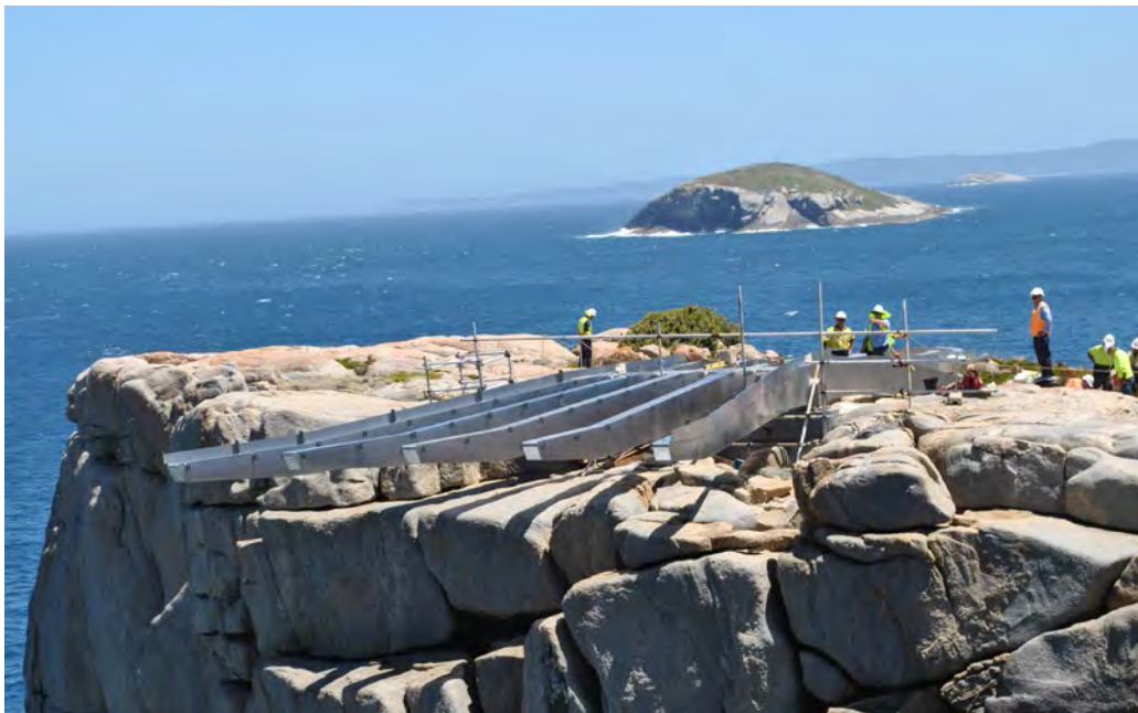
Cantilevered beams supporting The Gap lookout. Photo – Mike Shephard/Parks and Wildlife
