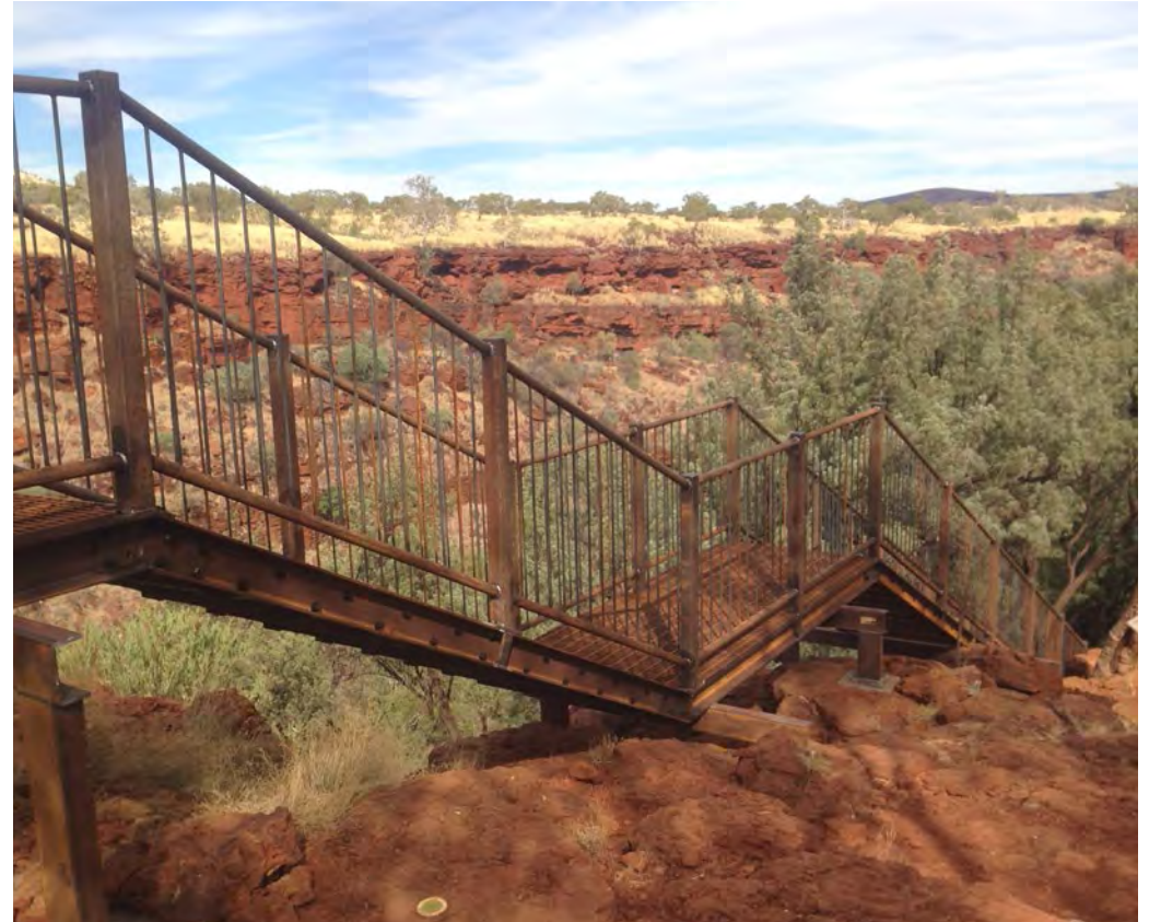
New walkway at Karijini National Park. Photo – Geoff Passmore/Parks and Wildlife
