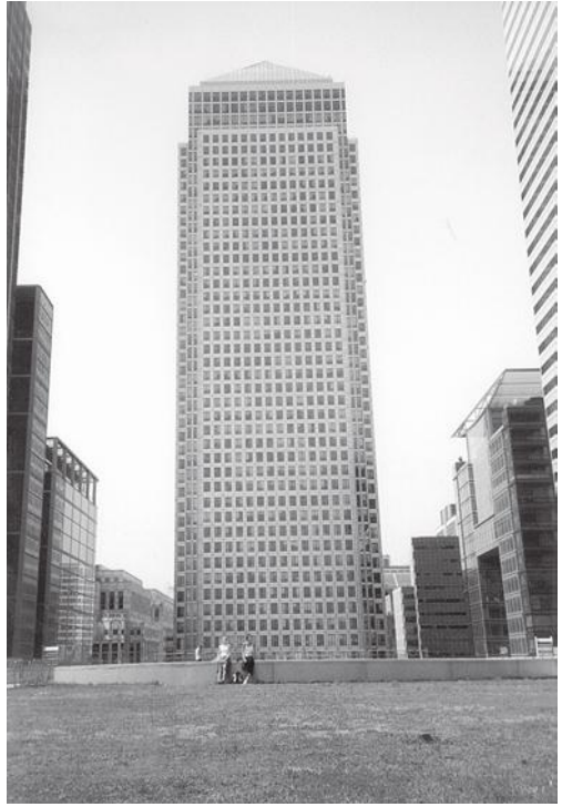
FIGURE 13. A living roof on top of a fifty-story building at Canary Wharf in Central London. Photograph by the author.
